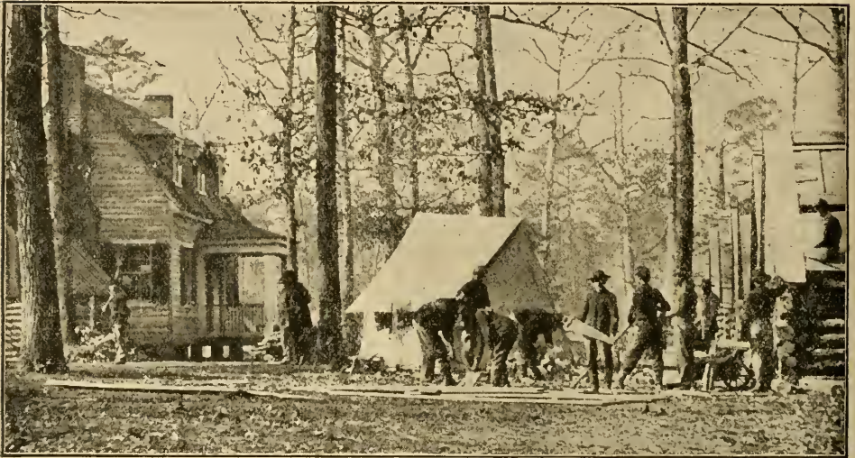
BUILDING CABINS FOR THE WINTER.
